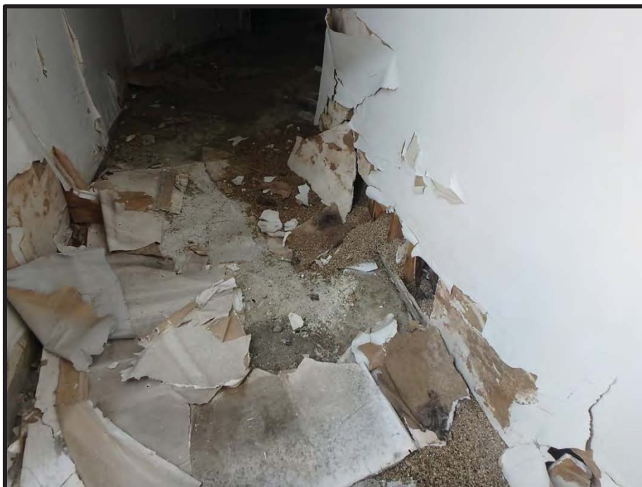
REPRESENTATIVE INTERIOR VIEW ASSUMED ASBESTOS CONTAINING VERMICULITE AND ASSOCIATED DEBRIS
