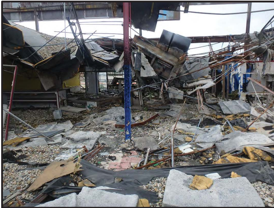
REPRESENTATIVE INTERIOR VIEW FIRE DAMAGED AND COLLAPSED AREA
