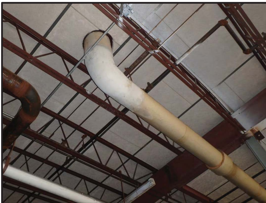
REPRESENTATIVE INTERIOR VIEW ASSUMED ASBESTOS CONTAINING THERMAL COMPONENT
