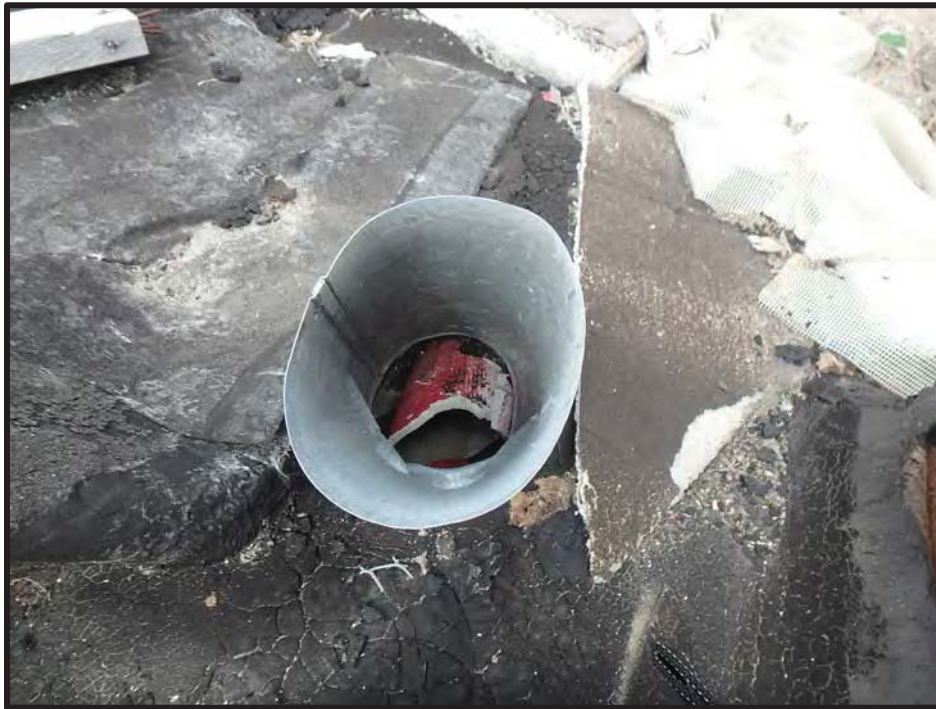
REPRESENTATIVE INTERIOR VIEW ASBESTOS CONTAINING TRANSITE PIPE AND ASSOCIATED DEBRIS
