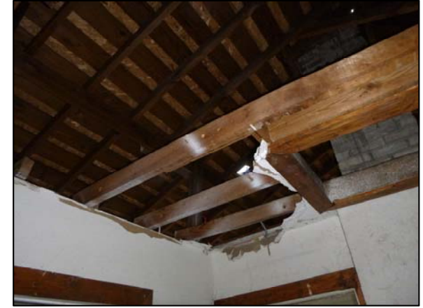
Vermiculite Insulation Throughout Removed
