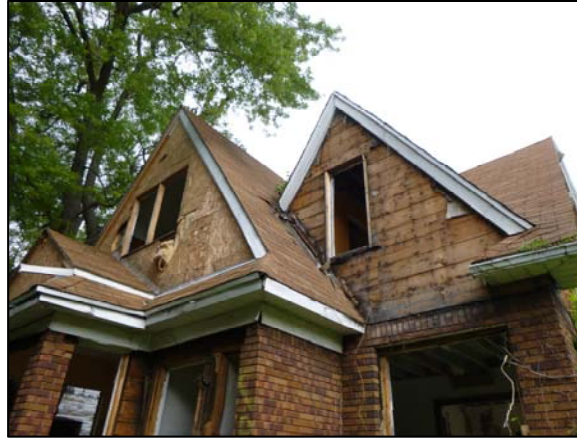
Exterior Stucco Exterior of House (top portion – under vinyl siding) Removed
