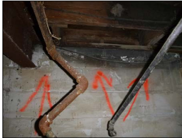
Duct Wrap (2" Tape) Basement Duct Work Removed
