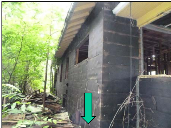
Black Exterior Caulk Back Right of House on Pipe Removed
