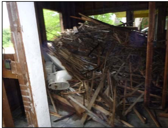
Joint Compound (Composite of Drywall and Joint Compound <1 % ACM) Throughout Removed
