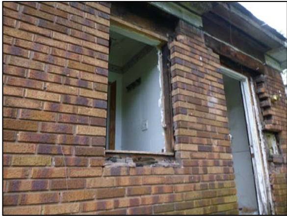
White Silicone/Beige Caulk Back Entry – Door Frame Removed
