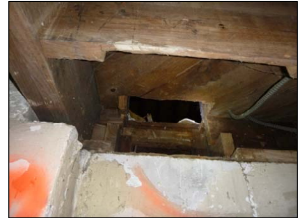
Duct Wrap (2" Tape) Basement Duct Work Removed
