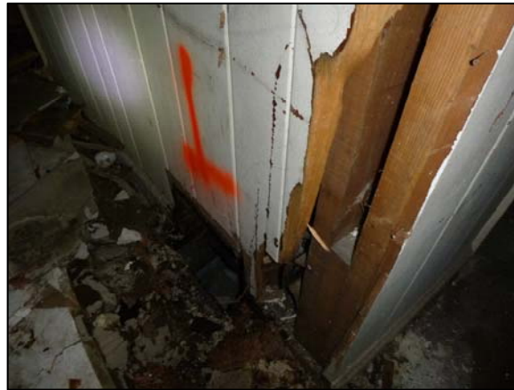
Duct Packing Register Boots Throughout Removed
