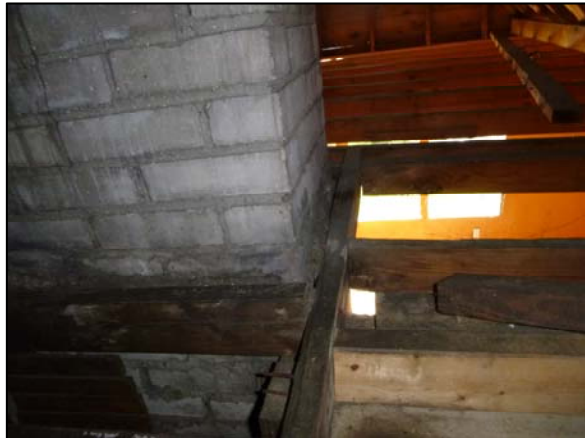
Vermiculite Insulation Throughout Removed
