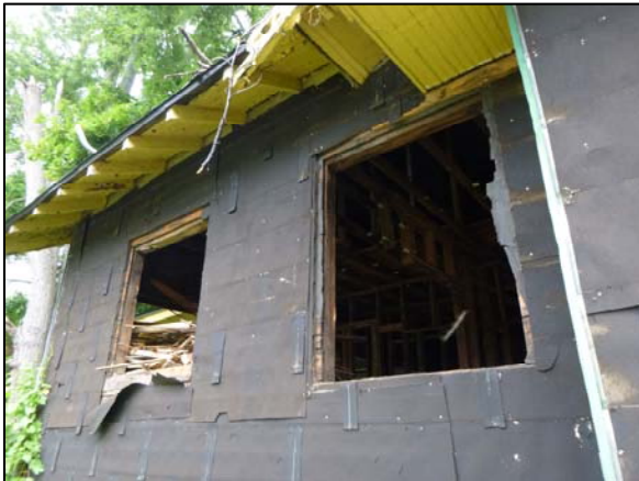
Window Glazing Windows Throughout Removed
