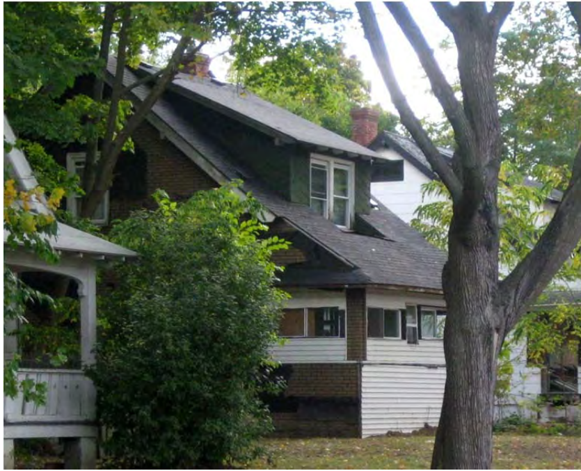
2314 Proctor Ave. Insensitive porch enclosure with incorrect siding; vinyl windows.
