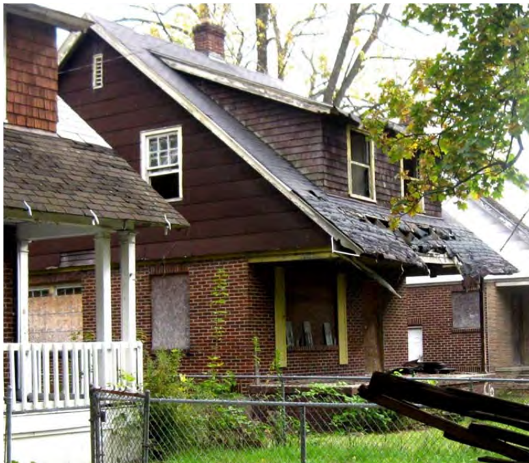
2338 Humboldt Ave. Missing porch supports; missing fenestration; damage to roof is substantial to becoming an integrity issue.
