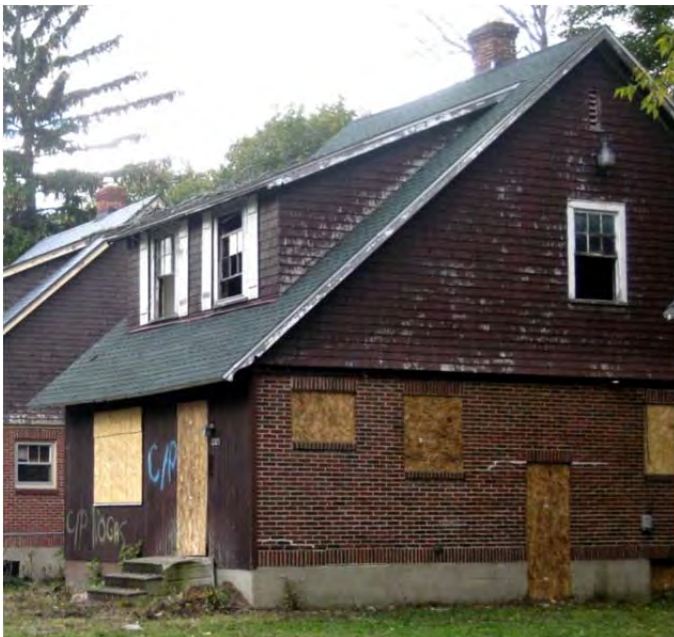
2321 Forest Hill Ave. Insensitive porch enclosure with T1-11 type siding at the front elevation.
