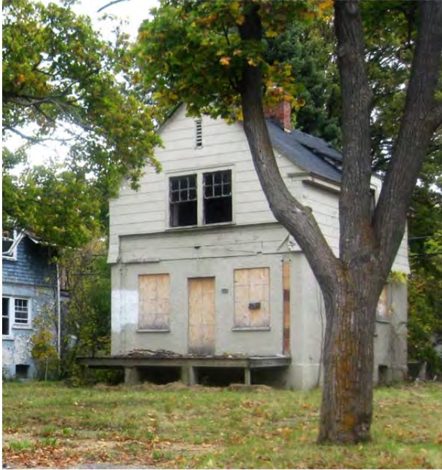
2638 Lawndale Avenue. Missing porch, missing steps, missing fenestration and door.
