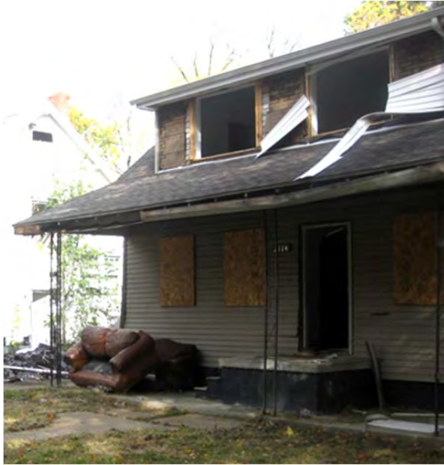
2114 Proctor Ave. Insensitive siding, missing siding, porch alterations, missing fenestration and door.
