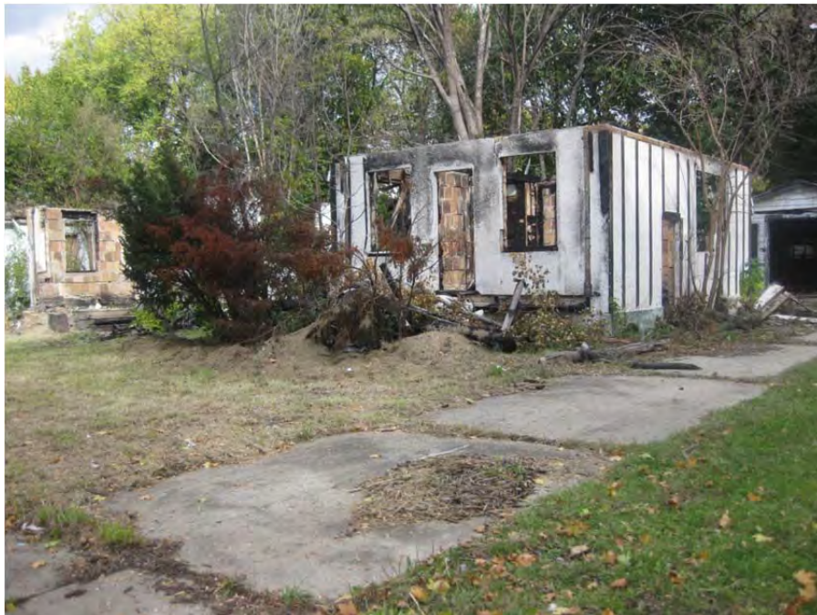
2122 Lawndale Ave. Substantial fire damage has severely compromised integrity.
