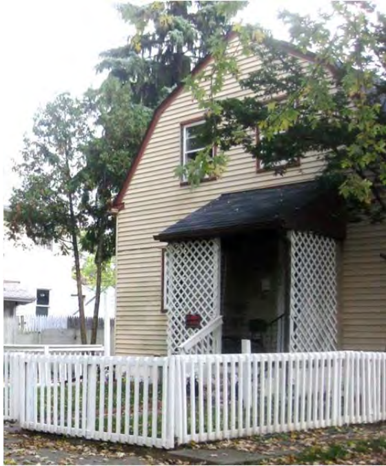
2302 Milbourne Ave. Recent siding is insensitive to original design; latticework at entry is recent; loss of smaller-scale design features upon elevations.
