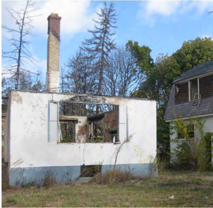
1222 W. Rankin St. Substantial fire damage has severely compromised integrity.
