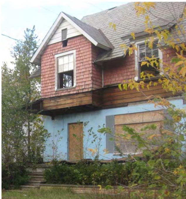
810 W. Paterson St. Missing porch, missing siding, missing fenestration, missing door.
