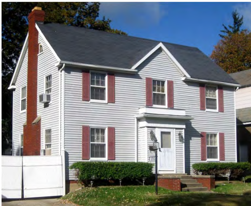
1713 Mt. Elliott. All-over siding; enclosed entry appears to be a later alteration.
