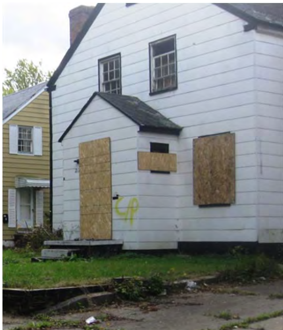
2121 Milbourne Ave. Insensitive siding, missing fenestration, entry bay appears to be substantially altered.
