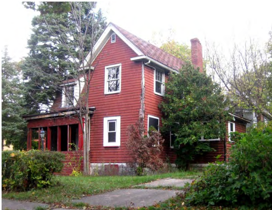
917 W. Dayton St. Faux ground floor windows.
