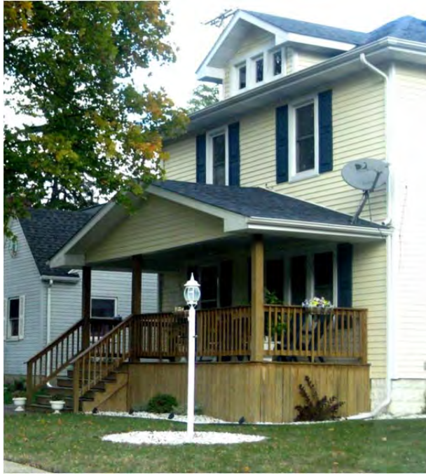
1906 Lloyd St. Porch appears to be reconstructed; boxed eaves appear to be more recent.
