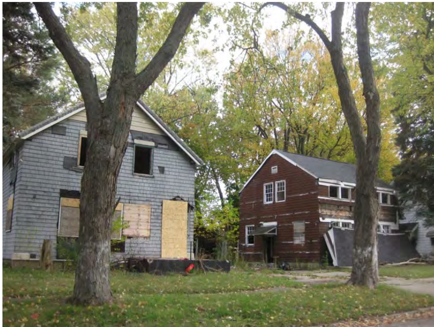
2132 and 2126 Milbourne Ave. 2132: missing entry, missing stairs, missing fenestration and door. 2126: collapsed porch, missing fenestration.
