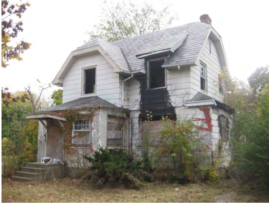
901 W. Paterson St. Missing fenestration, altered eaves, siding appears to be incorrect in conjunction with stucco entry, which itself may be an alteration.
