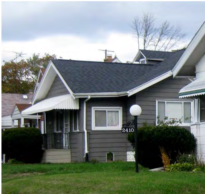
2414 Bassett Pl. New siding that appears to be synthetic or metal; vinyl or metal frame windows, elevated entry appears compromised with new materials.
