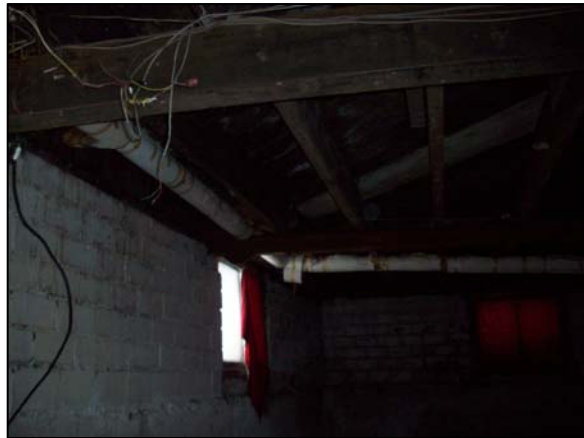
Mag Straight Run and Mag Fittings Basement
