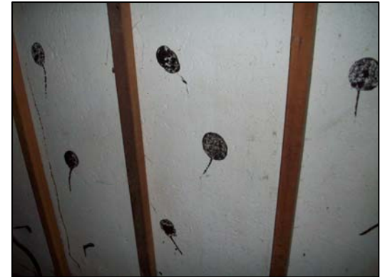
Glue Pad Basement Wall
