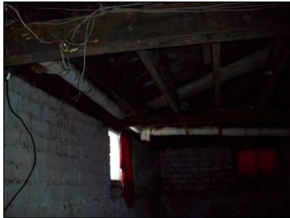
Mag Straight Run and Mag Fittings Basement
