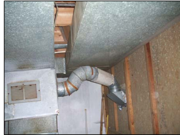
Example of Duct Wrap Basement
