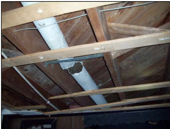
Example of Duct Wrap Basement
