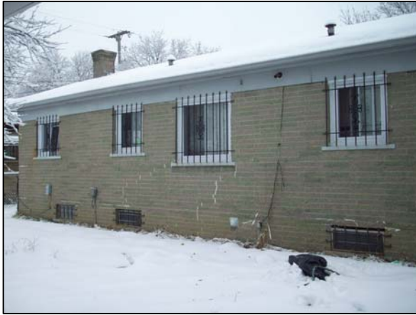
Example of Window Caulk Basement Windows
