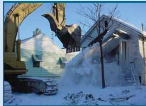
Genesee County Landbank's 500th Demolition
