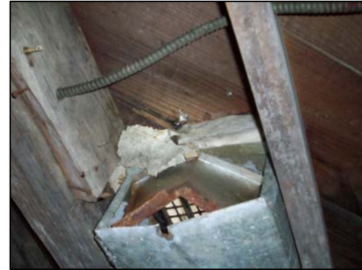
Example of Duct Wrap Basement
