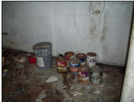
Paints and Sealer Basement
