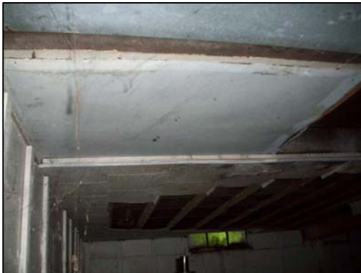
Example of Duct Wrap Basement
