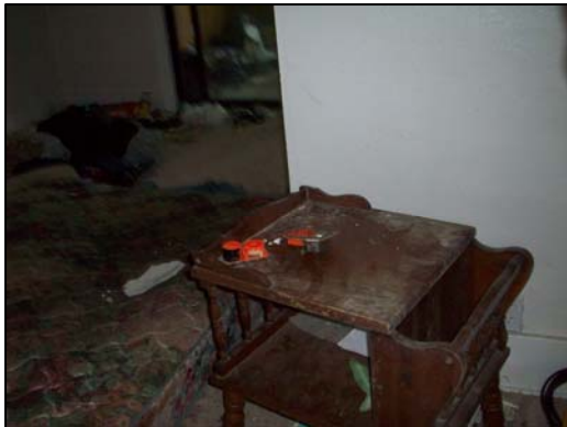
Smoke Detectors Living Room
