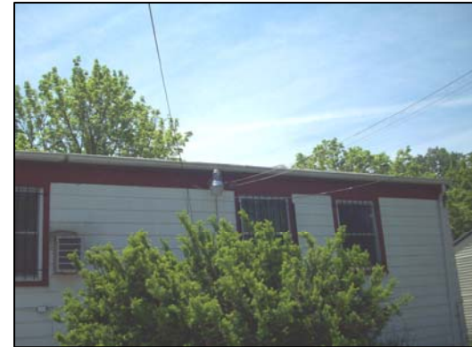
Mercury Light Back of House
