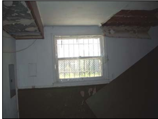
Window Caulk Basement Windows
