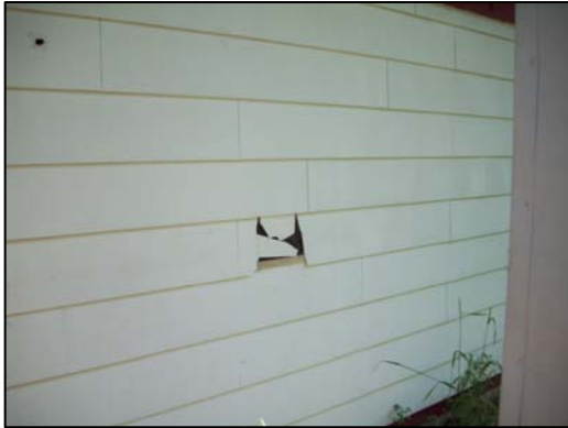
Transite Siding Exterior Siding
