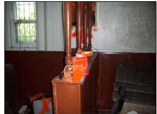
Battery and Smoke Detector Basement
