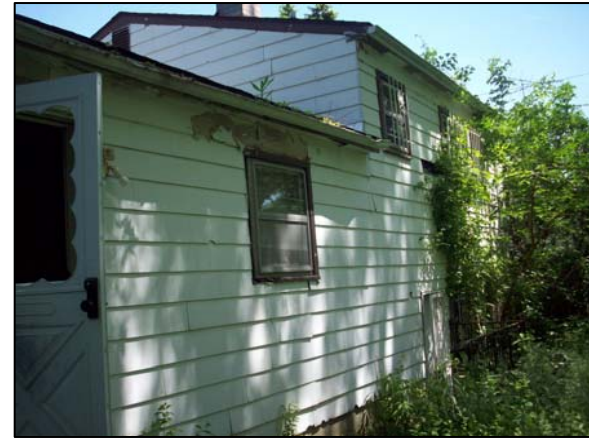
Example of Transite Siding Exterior Siding
