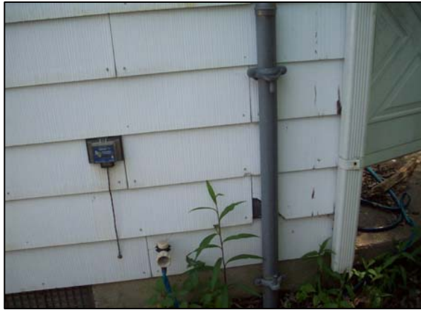
Example of Transite Siding Exterior Siding
