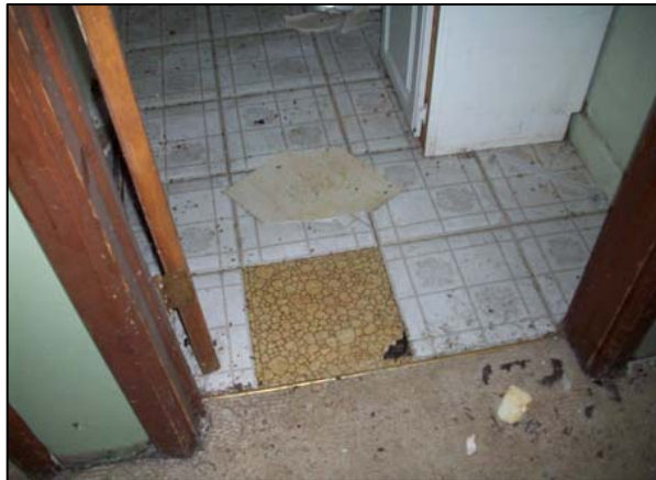
Linoleum Yellow Pebble Pattern and Black Mastic Throughout Basement
